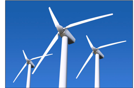
Windmill Blade Repair & Epoxy Curing
